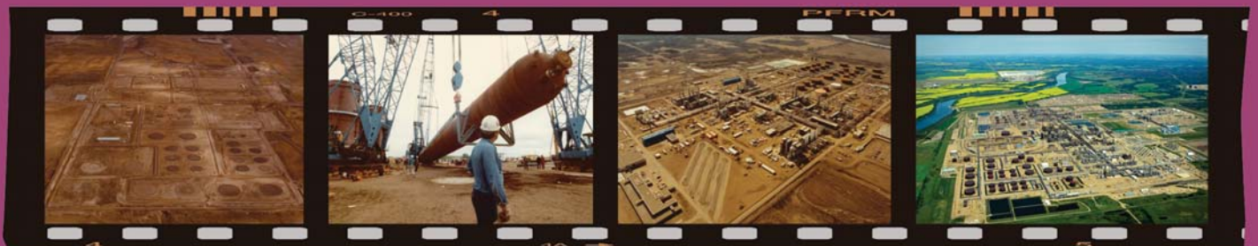
October 1981, early construction at Scotford Refinery.
