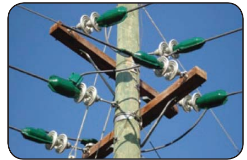
The new moulded covers help protect birds from electrocution.
